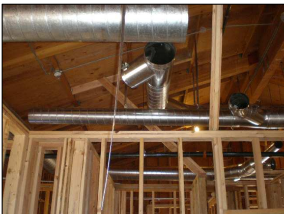
Installing HVAC and Fire Sprinkler Systems
