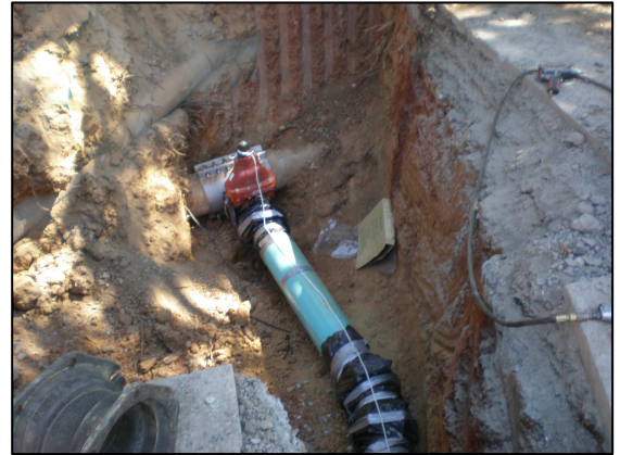
Installing New Fire Hydrant
