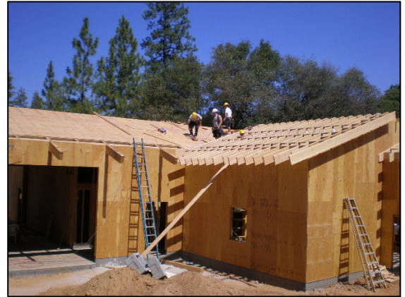
Installing Roof Sheathing
