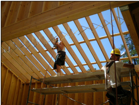
Installing Tension Straps
