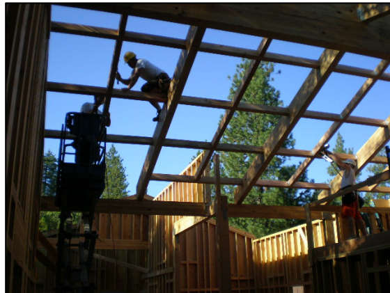
Framing Roof at New Building Addition
