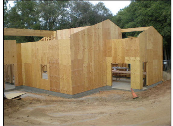
Framing exterior walls
