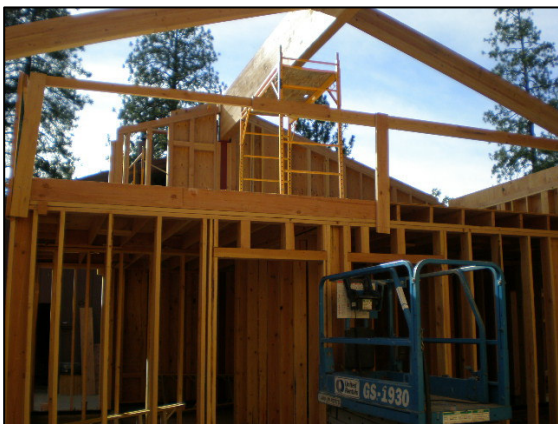
Framing interior walls
