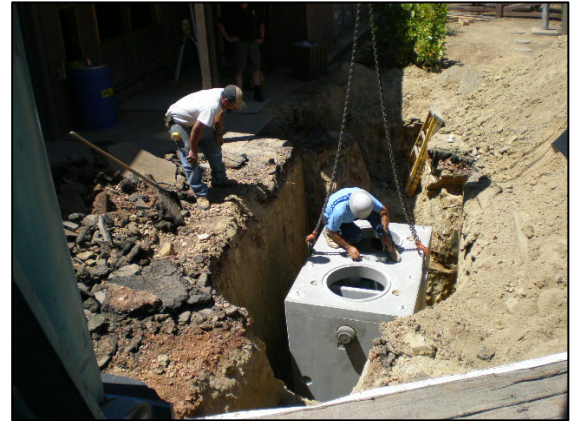
Installing the sand/grease separator
