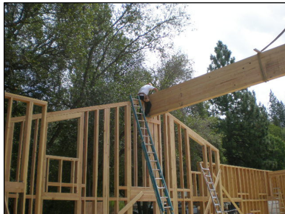
Setting Glue Laminated Beams
