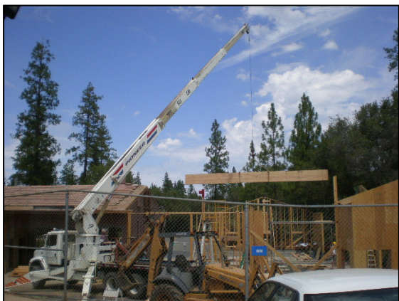
Setting GL Beams
