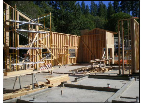
Framing Exterior Walls at Addition
