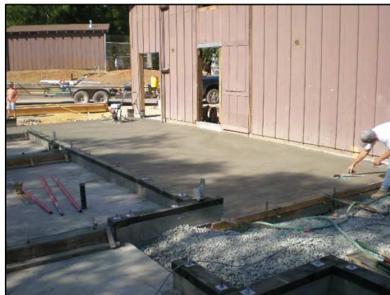
Finishing Slab at New Apparatus Bay
