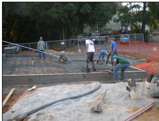
Pouring Foundation Slab at the East Side Addition
