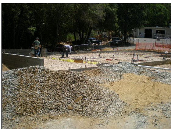
Installing Slab Bedding & Rebar
