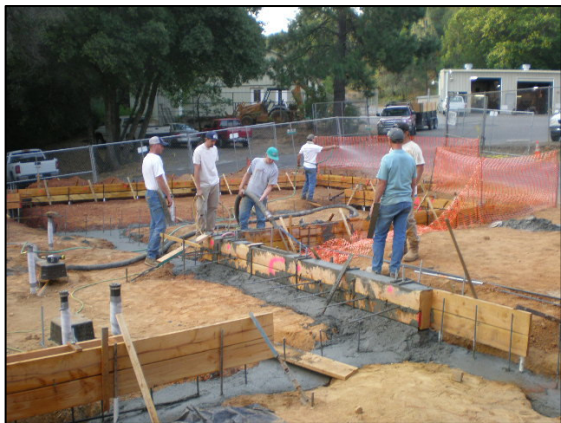
Pouring Concrete for Footings & Curbs
