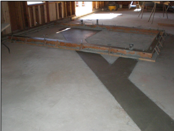
Repairing/Patching Existing Floor
