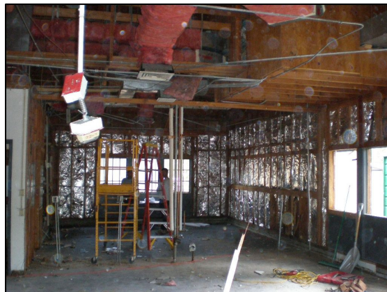
Demolishing Walls and MEP Systems
