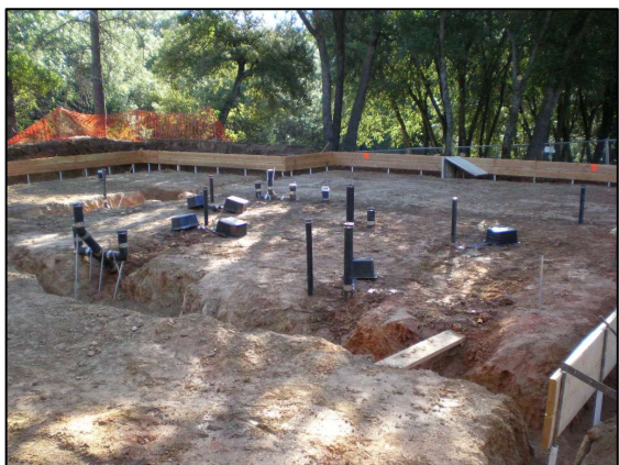
Installing Sub Grade Plumbing
