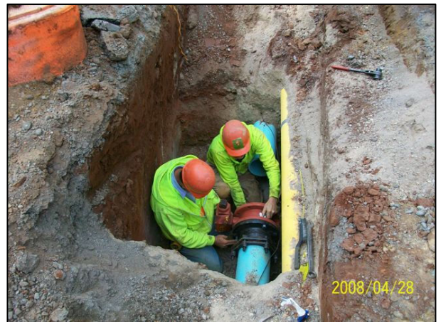
Installing 8" Water Valve
