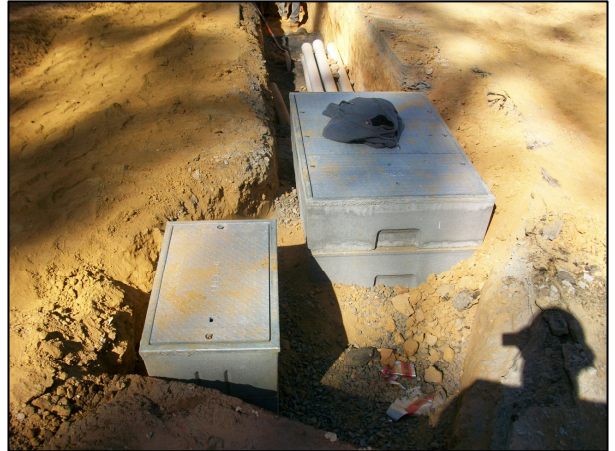
Installing Electrical Pull Boxes
