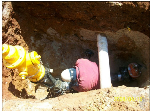
Installing Fire Hydrant
