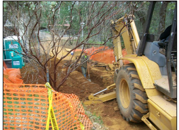
Excavating Fire Water Trench at Building "C"
