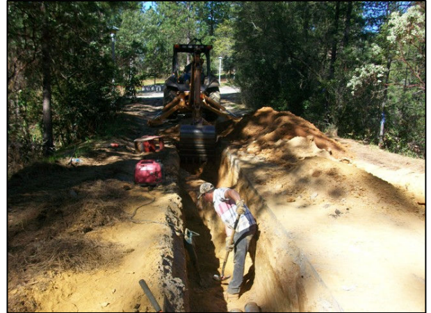
Excavating Electrical Trench East of Toyon
