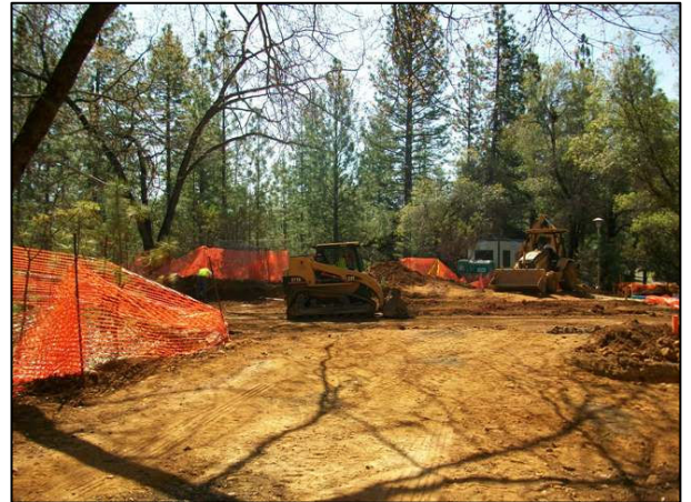
Cutting Pad for Building "C"
