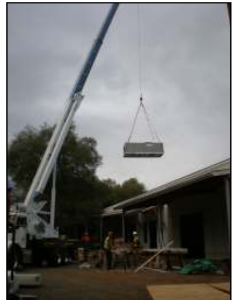
Installing HVAC Unit
