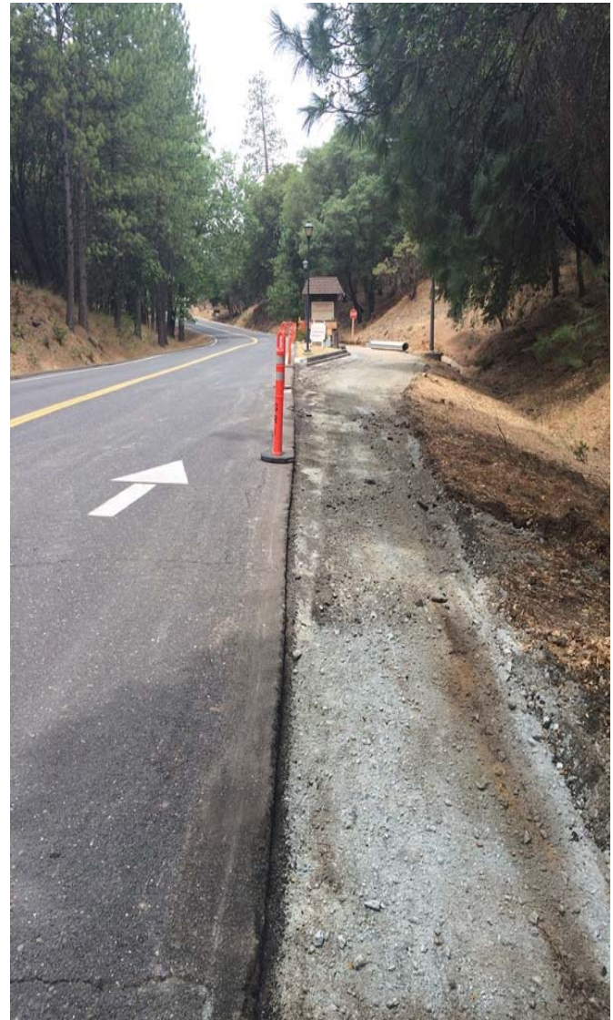
Demo work at the information booth
