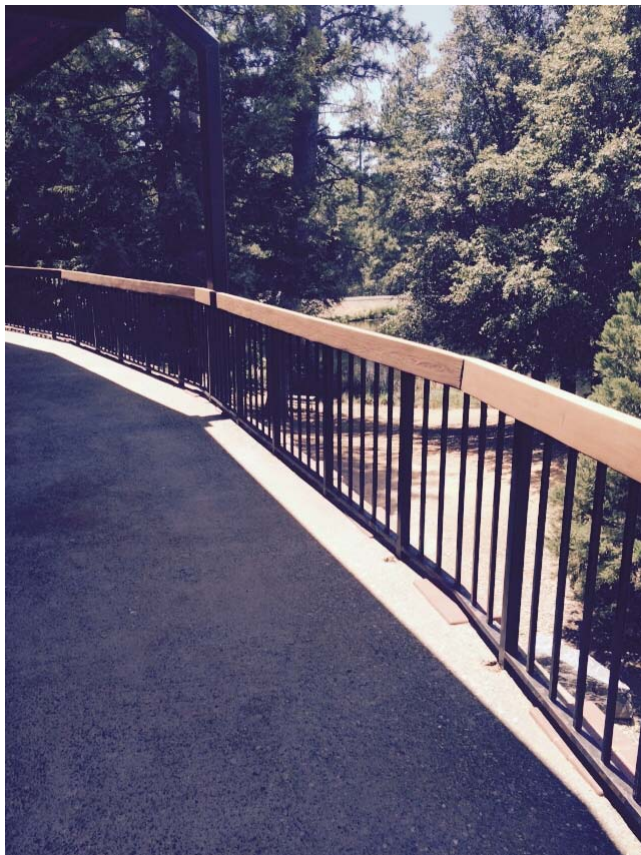
Wood sanding @ upper level railing
