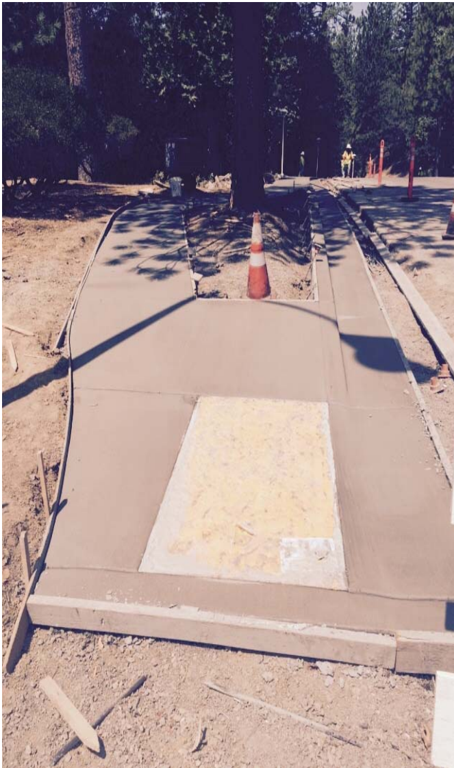
Sidewalk @ the fire house
