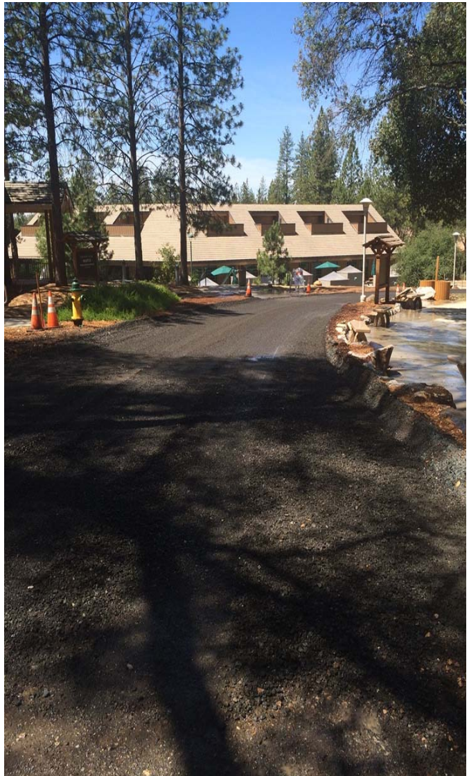
Graveling & Compaction (Front of Child Care)
