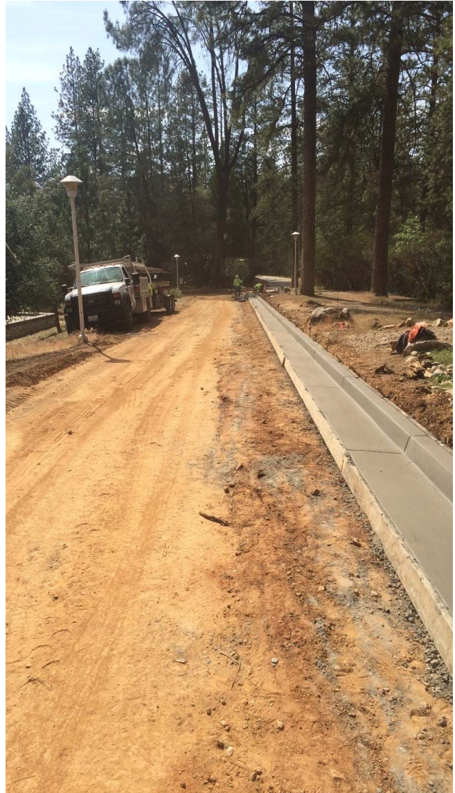
Curb & gutter (From Pinyon to Sequoia)
