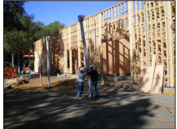
Setting exterior steel columns
