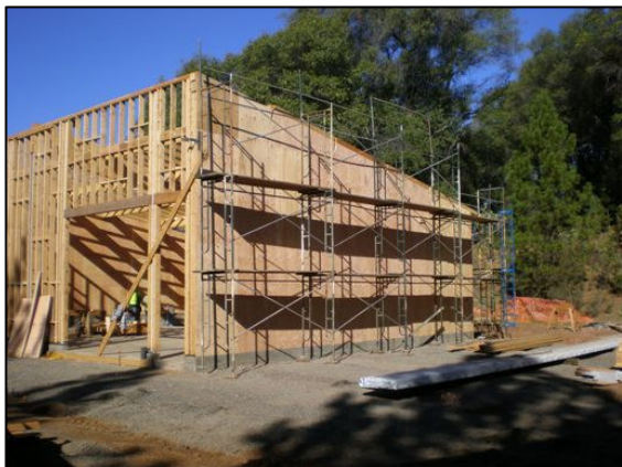
Erecting scaffolding
