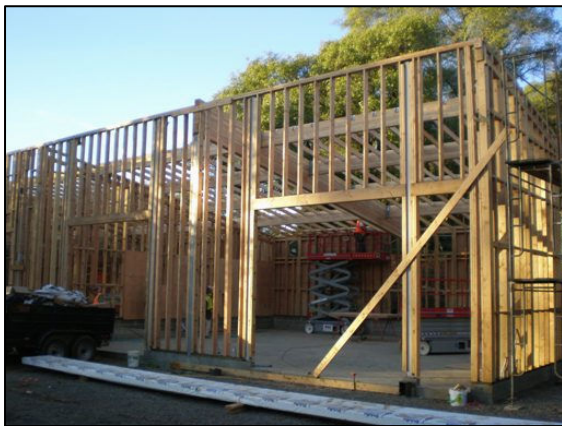
Framing exterior walls and roof
