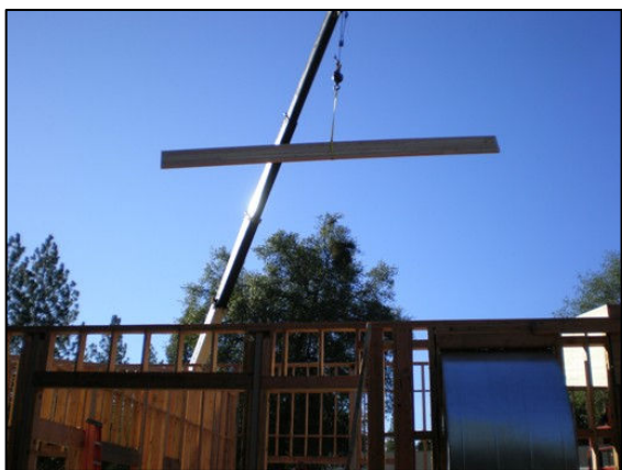
Installing the glue-laminated beams
