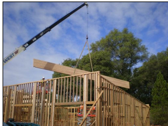
Installing the glue-laminated beams
