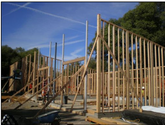
Framing exterior walls and installing steel columns
