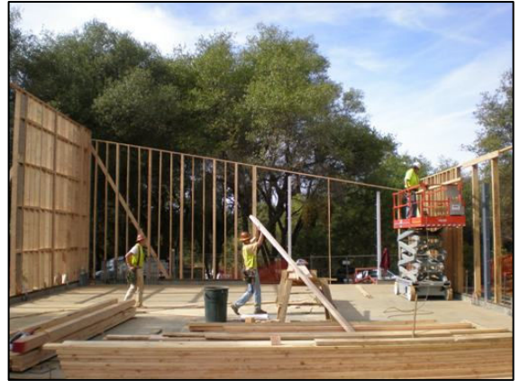
Framing exterior walls
