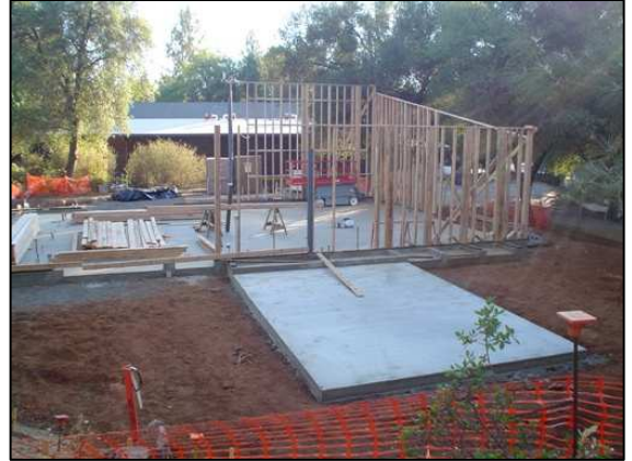
Framing exterior walls
