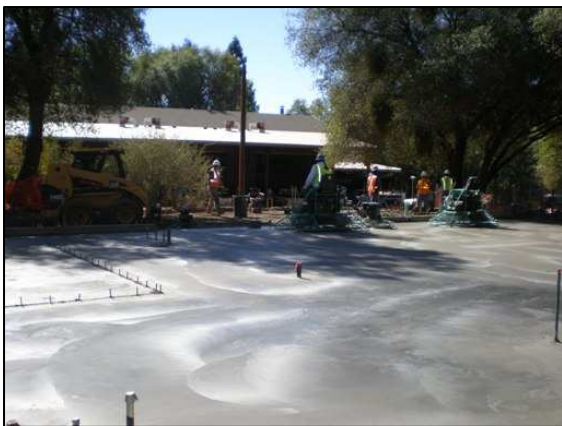
Finishing slab
