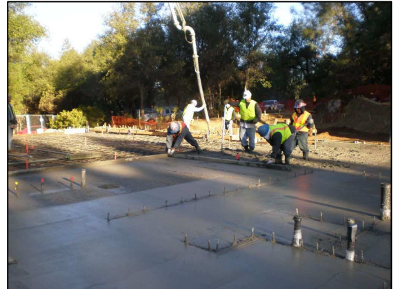
Pouring slab on grade
