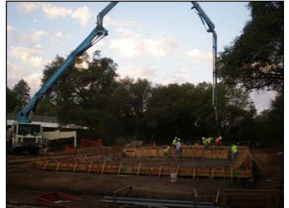
Pouring footings, curbs and stem walls
