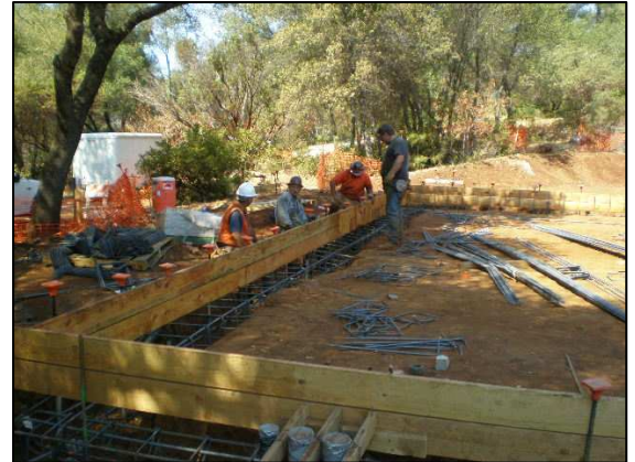
Installing reinforcing steel
