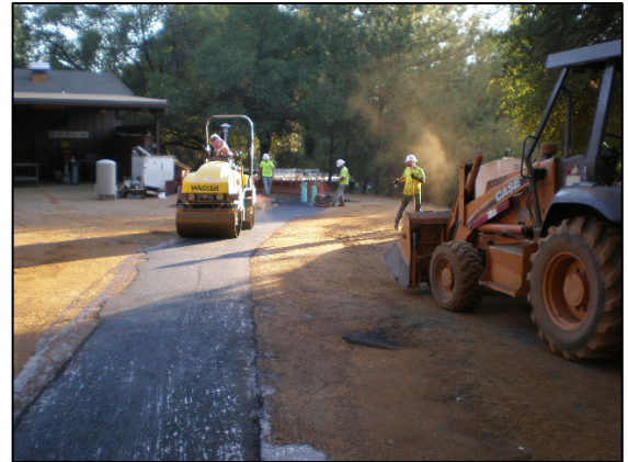
Paving Joint Utility Trench
