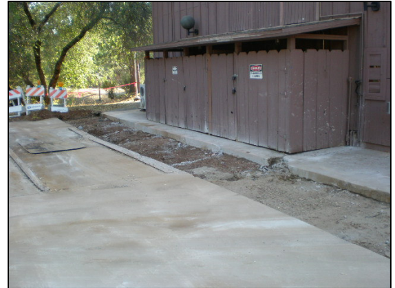
Saw cutting existing paving for new telecommunications trench
