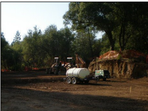
Grading building pad
