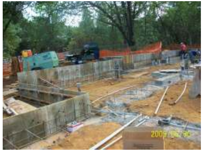
Form Stem Walls at Building "C"
