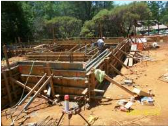
Place Under Slab Utility Rough-ins at Building "B"
