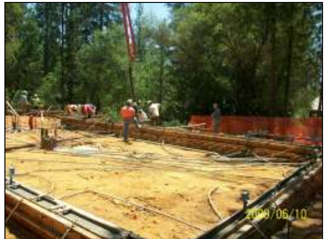
Placing Stem Wall Forms & Concrete at Building "E"
