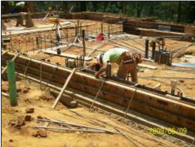
Placing Stem Wall Forms & Concrete at Building "E"
