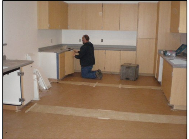
Installing Casework
