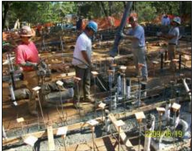
Placing Concrete at Building "C"
