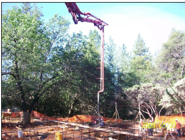
Placing Concrete at Building "B"
