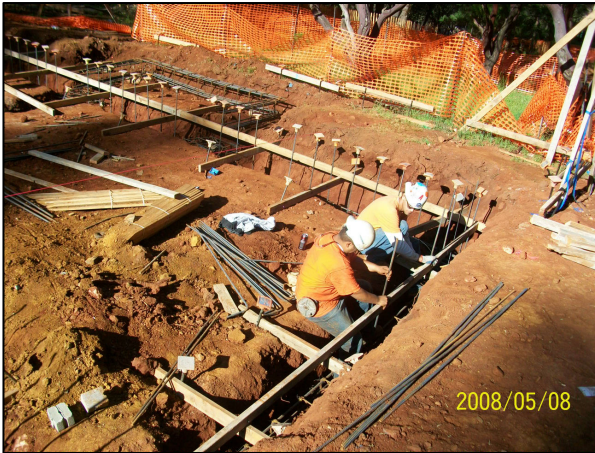
Installing Rebar at Building "B"
