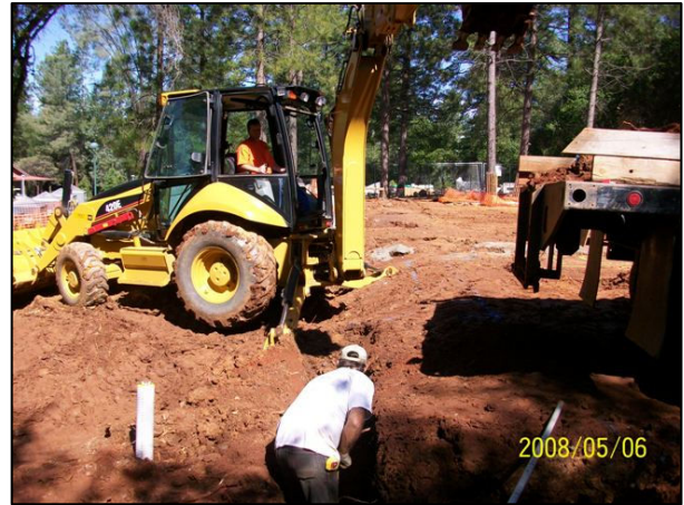
Excavating Footing Trenches at Building "E"
