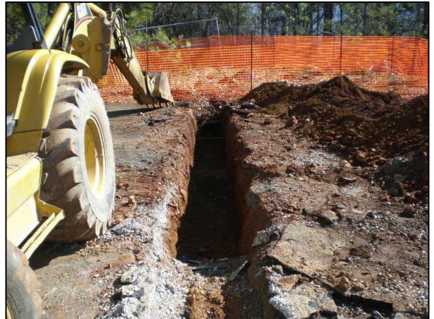
Installing Site Utilities
