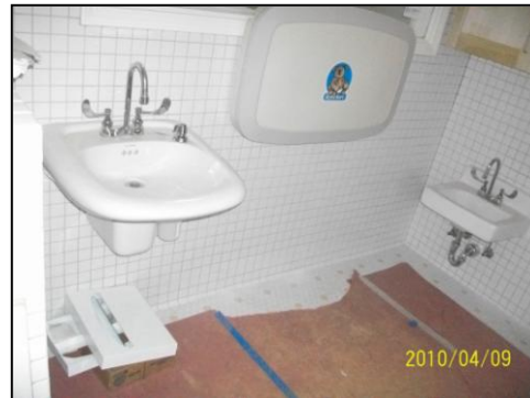
Interior finishes installation in progress, adult sink, child sink, diaper changing table
