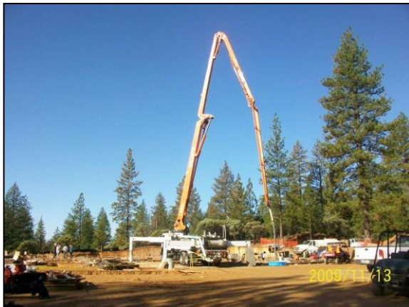
Concrete pump truck setting up for concrete placement
