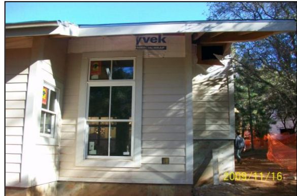
Building "E" exterior siding installation in progress
