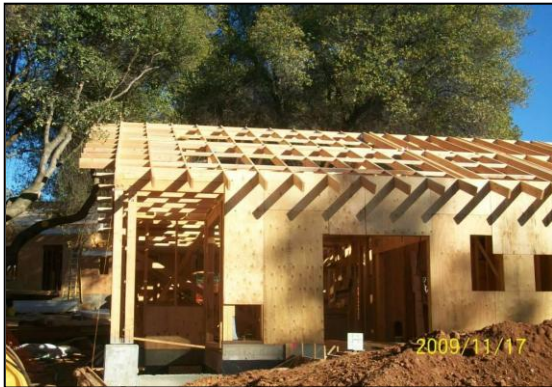
Building "A" roof framing in progress
