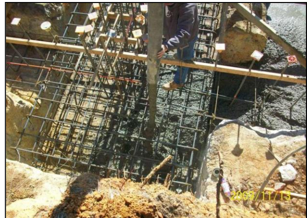
Placing concrete at Building foundation in progress
