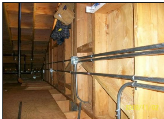
Building "B" interior electrical installation in progress
