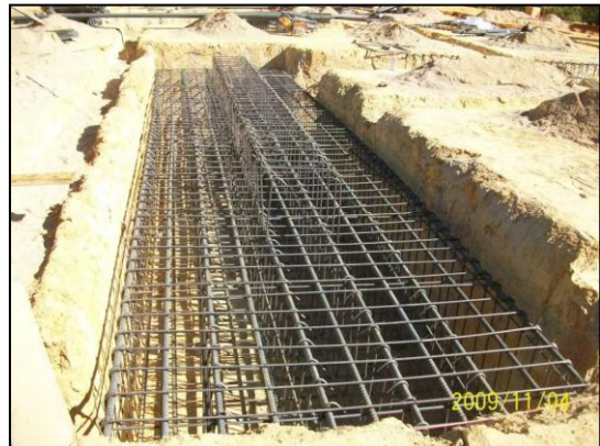
Begin installation of Building foundation reinforcing
