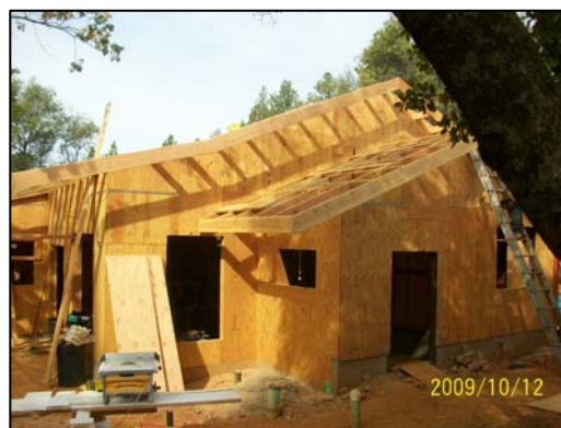
Building "B" roof framing in progress
