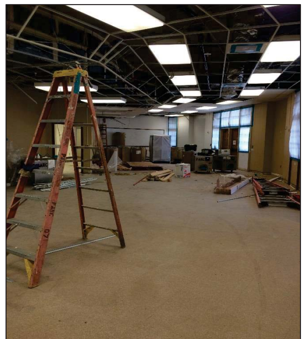
Lower Manzanita – Non Hazardous Remediation Ceiling Grid
