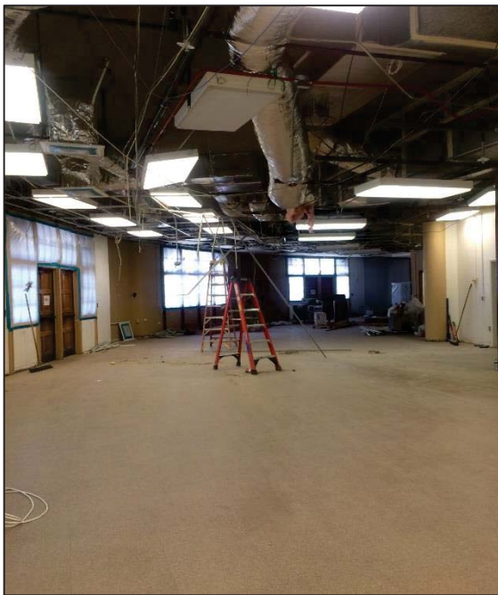
Lower Manzanita – Non Hazardous Remediation Ceiling Grid
