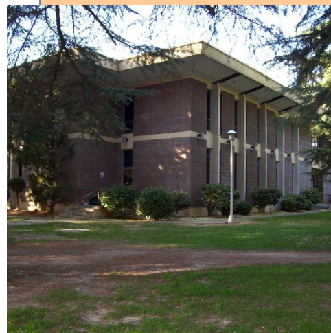
Morris Bldg at MJC East Campus
