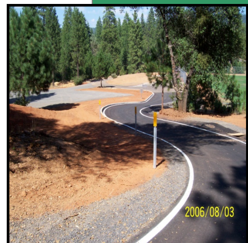
New Secondary Access Road
