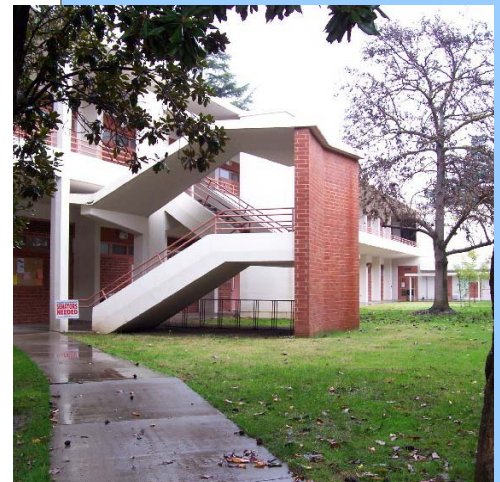
Existing Science Building at East Campus
