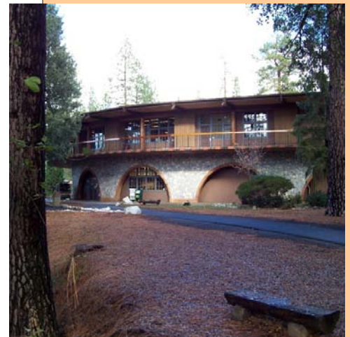
Manzanita Bldg at Columbia College
