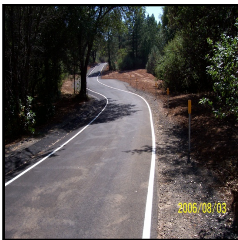
New Secondary Access Road
