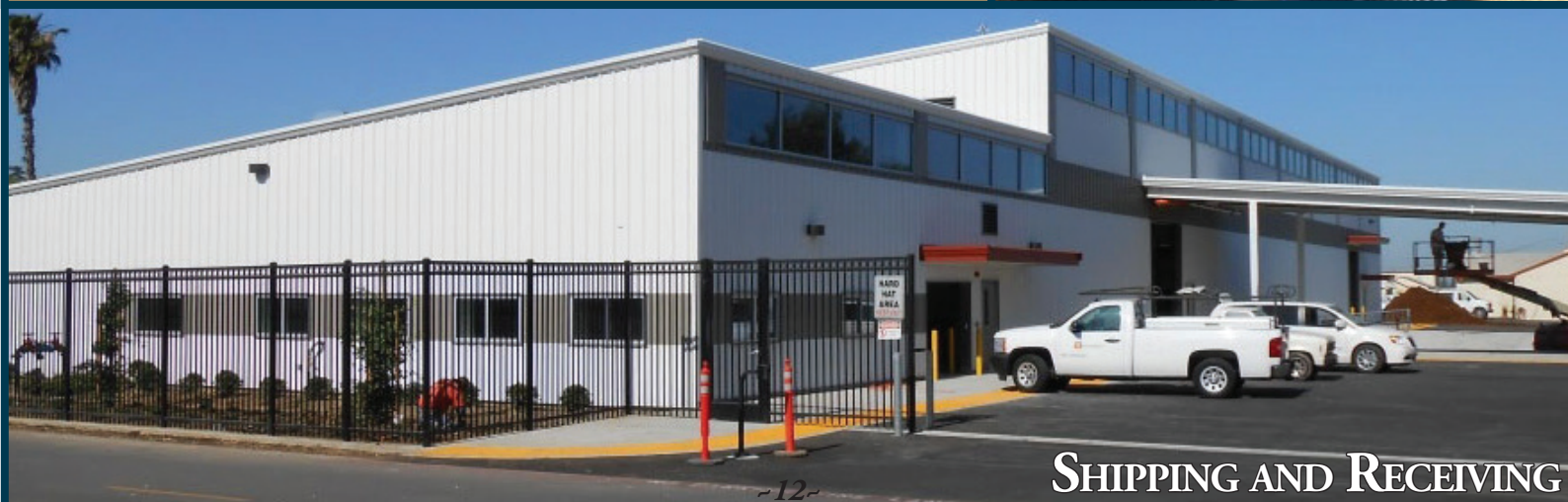
SECONDARY DATA CENTER
