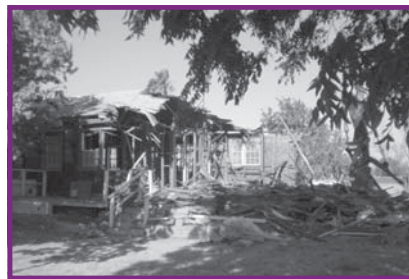
Demolition of current modular Ag units, MJC
